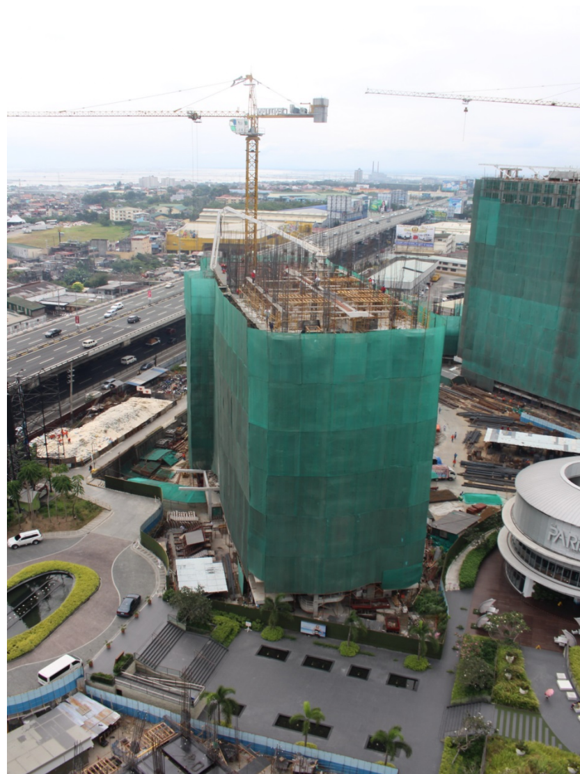
Concrete Pouring for Maldives' 15 th floor is ongoing.
